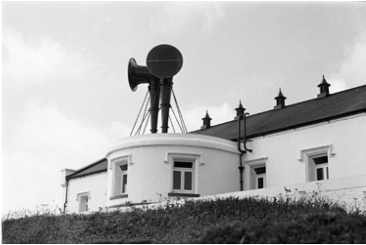
ABOVE LEFT: Two large black trumpets were used for the fog signal at the Lizard lighthouse and these remain in place today, along with the machinery used to make the signal.
