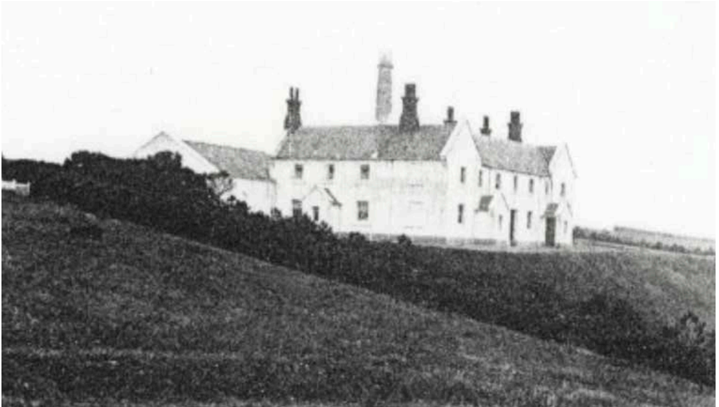
ABOVE: By the 1860s, South Foreland had become one of the most significant lighthouse stations in the Trinity House jurisdiction. As the site for the development of cutting-edge technology, it required the construction of new buildings, an engine house, more accommodation and even pig sties.
